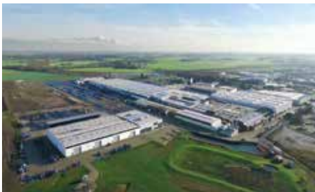
State-of-the-art, 592,000-sq. ft. Factory and Head Office in Alpen, Germany
